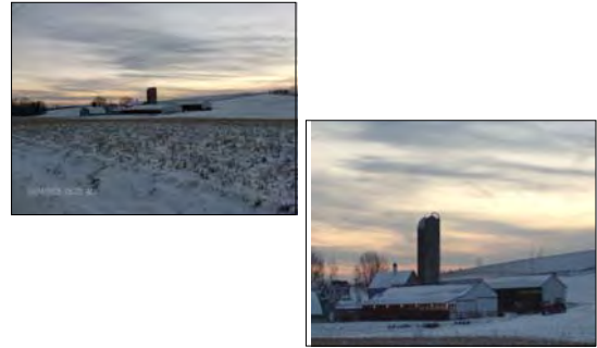
Schlegel Dairy Freestall
