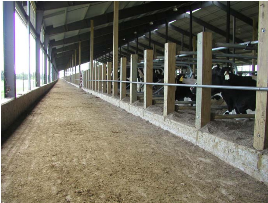
Figure 3. A transfer alley used to move cows between pens in a well managed transition cow facility. Although the front of the stalls are open, note the deterrent bar which is located too low to allow cows freedom to lunge forwards in the stall.
